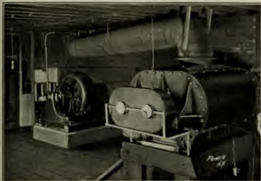
FIG. 2. BLOWER BELTED TO MOTOR
